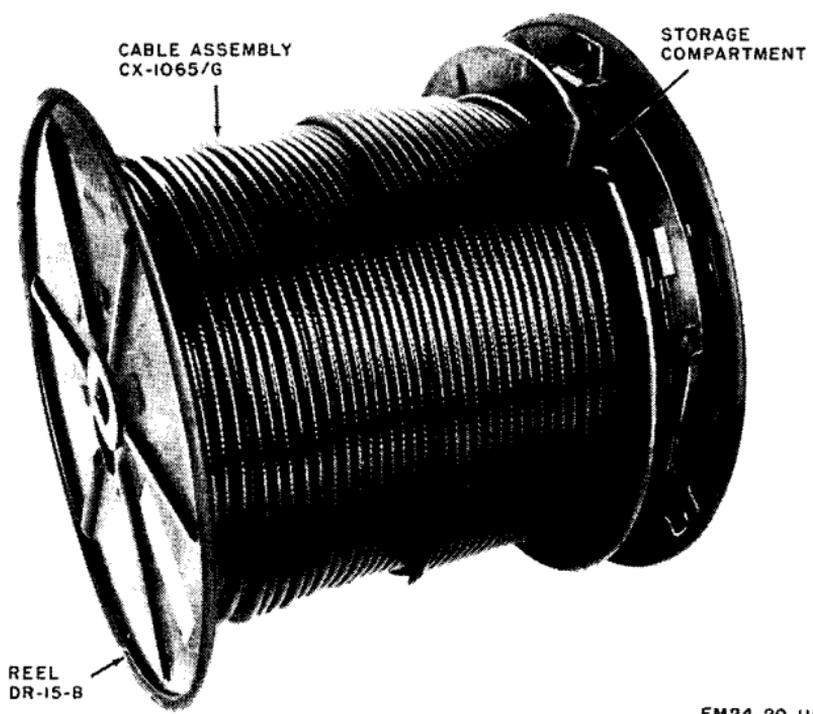
*Figure 7. Cable Assembly CX-1065/G, wound on Reel DR-15-B.*
