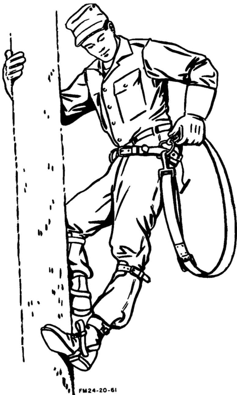
*Figure 71. Unhooking safety strap.*
