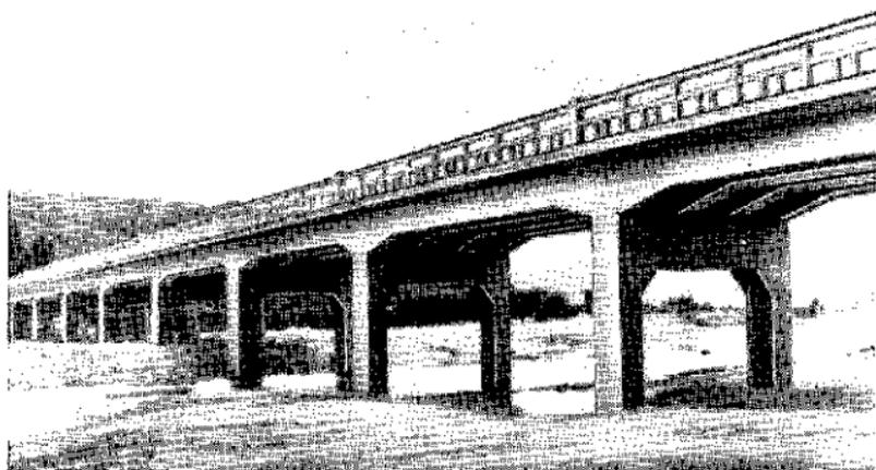
Figure 69. Typical multispan concrete T-beam bridge.
