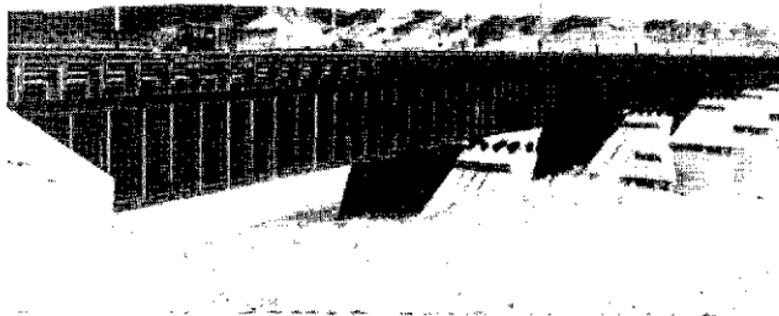
*Figure 78. Typical multispan plate girder bridge.*
