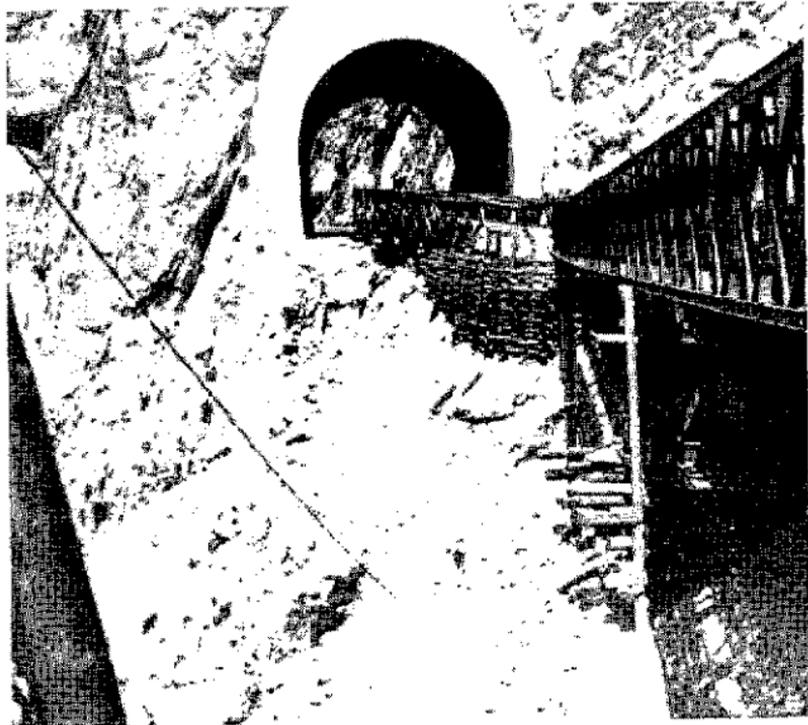
*Figure 123. Typical concrete tunnel portal.*
