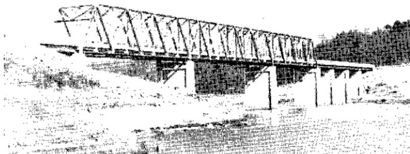
*Figure 75. Typical steel through truss bridge (Warren type).*
