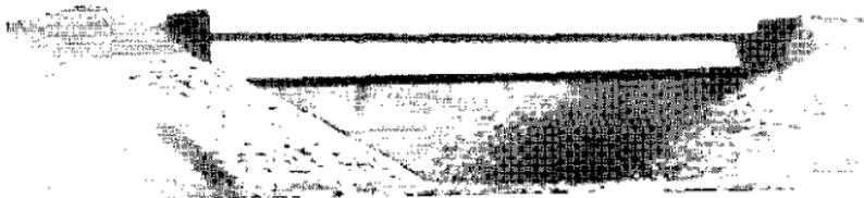
*Figure 66. Simple stringer bridge with steel I-beams and concrete slab flooring.*
