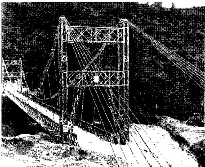
*Figure 91. Bailey type suspension bridge.*
