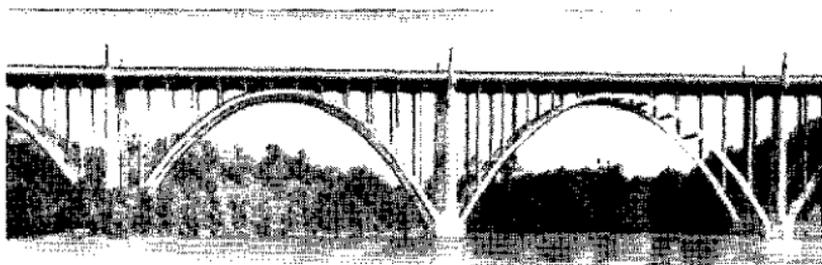
*Figure 87. Steel trussed deck arch bridge.*
