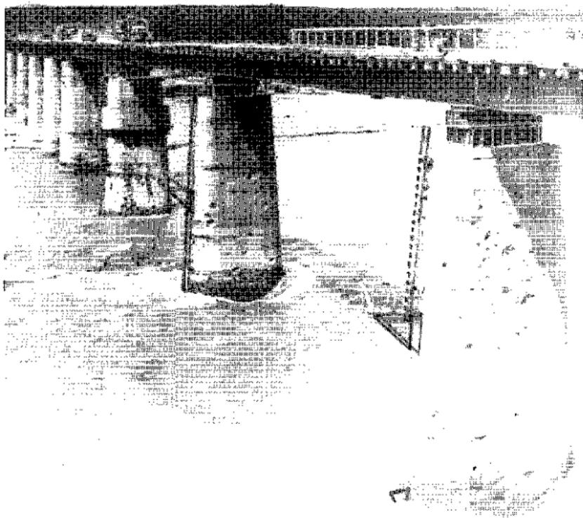
*Figure 103. Typical solid concrete pier.*
