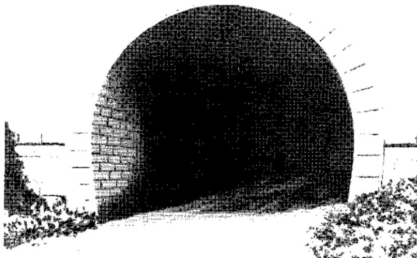
*Figure 120. Typical masonry lined tunnel.*
