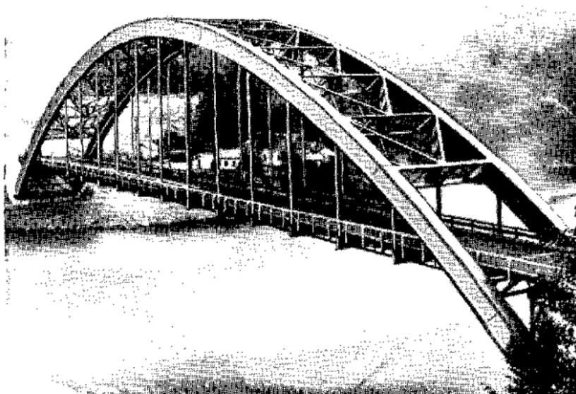
*Figure 88. Steel arch bridge, through type.*
