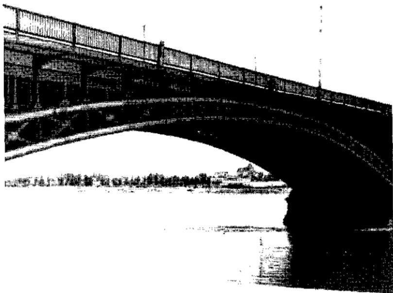
*Figure 86. Parallel curve, steel rib, arch bridge.*
