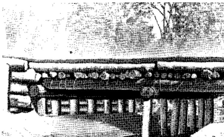
*Figure 64. Simple stringer bridge with log stringer.*
