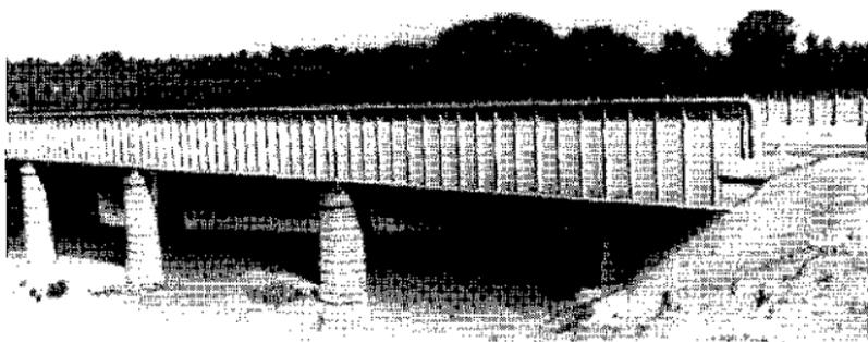
Figure 79. Through type girder bridge.
