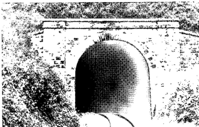
*Figure 122. Typical masonry tunnel portal.*
