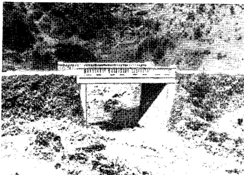
*Figure 67. Typical single span concrete bridge.*
