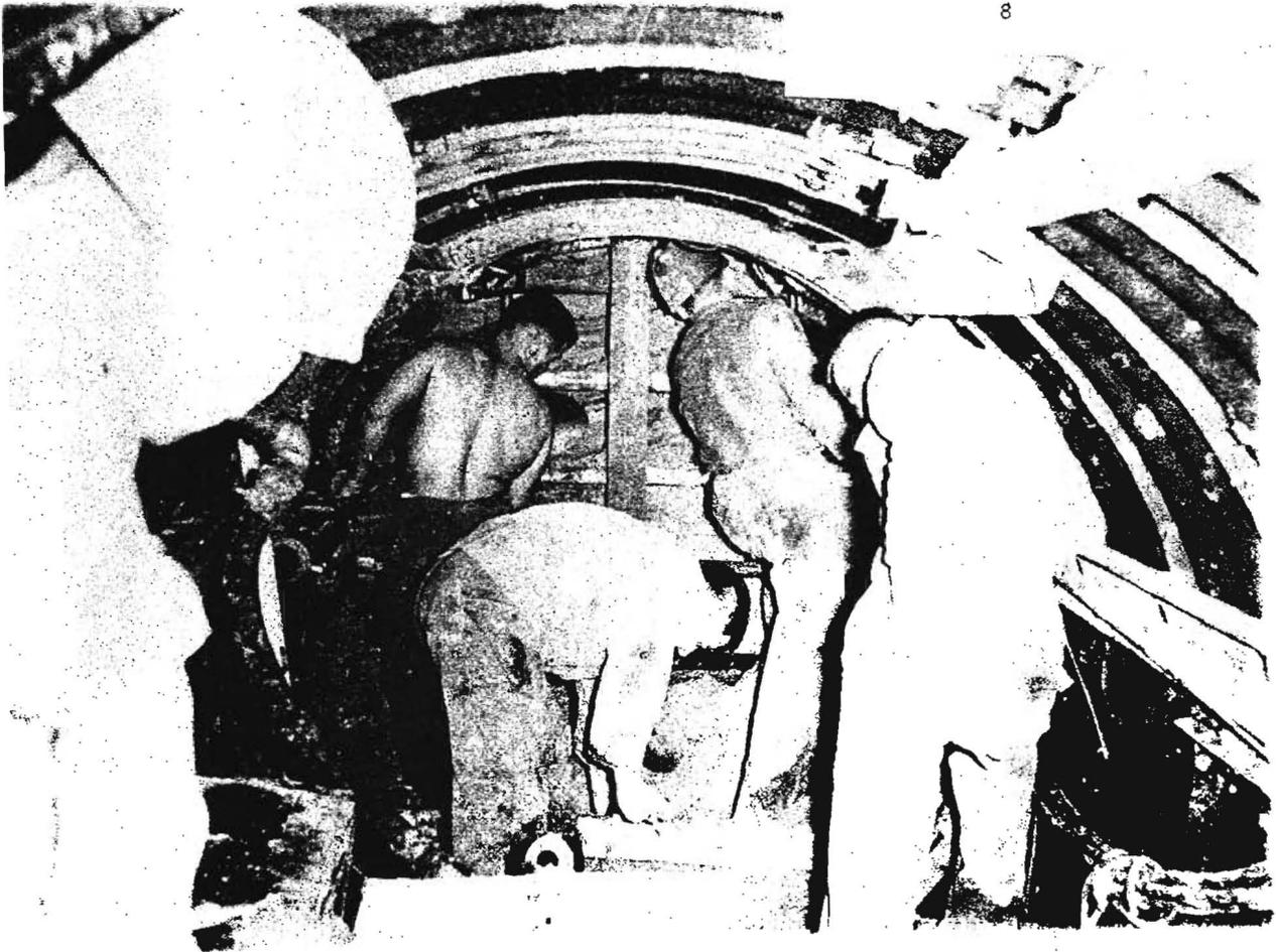
Figure 8 - Excavating Using the Blinds
