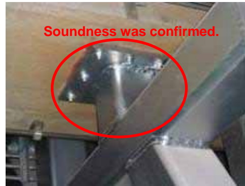
Pipe support structure
