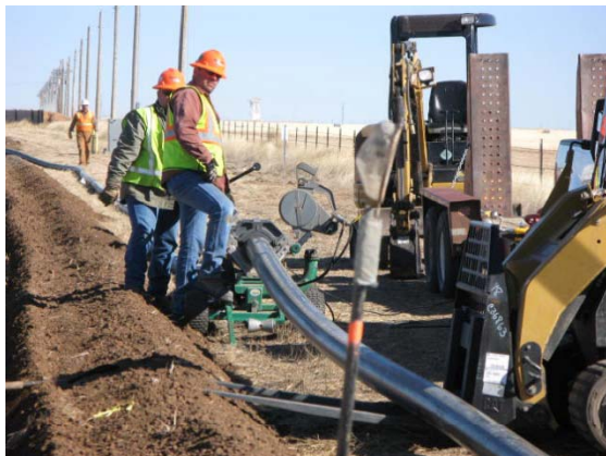
Installation of a conveyance line that transports treated water from the southeast pump & treat system to the Zone 11 ISB.
