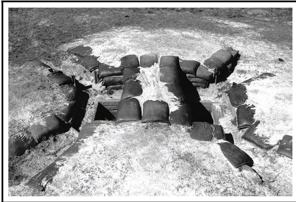
**Figure 6-15. Two-man fighting position with built-up OHC (Stage 4).**
