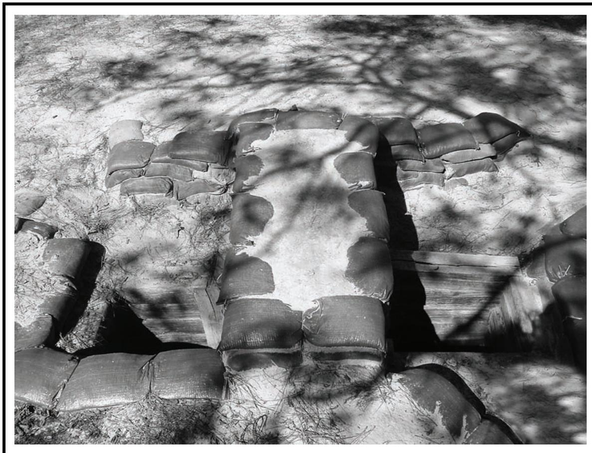
**Figure 6-20. Machine gun fighting position with OHC.**
