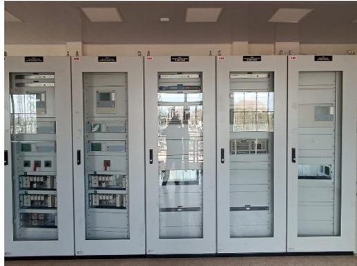
Fig. 1. A typical substation automation system cum communication panel
